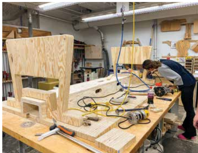
At top, a perspective rendering showing the Community desks on the third floor studio of the Anthony Timberlands Center. Above, student Emma Elkman works on the Community desk in the woodshop.
