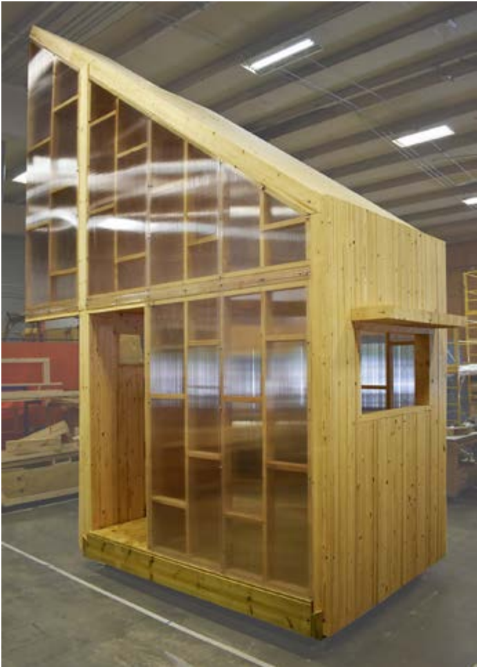
A view of the completed WLT assembly and framing.
