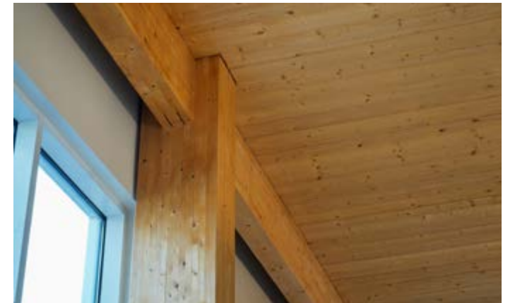
A detailed view of the mass timber used in Adohi Hall. Advanced timber technologies used for this structure include cross-laminated timber (CLT) panels and glulam beams and columns.
