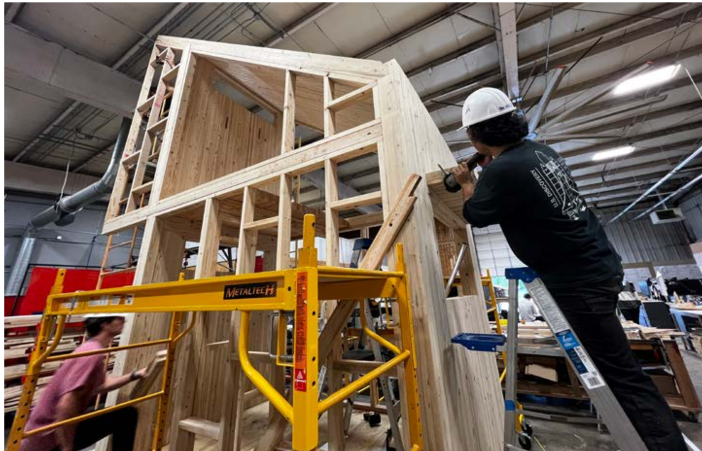
Josh Amaya, right, installs passive solar shading elements over a window on the full-scale mockup.
