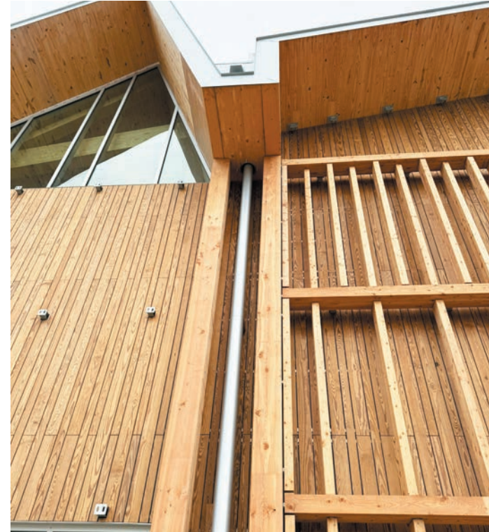
Rainwater caught by a "canoe" gutter is diverted by a downspout to gardens below. Photo by Modus Studio.
