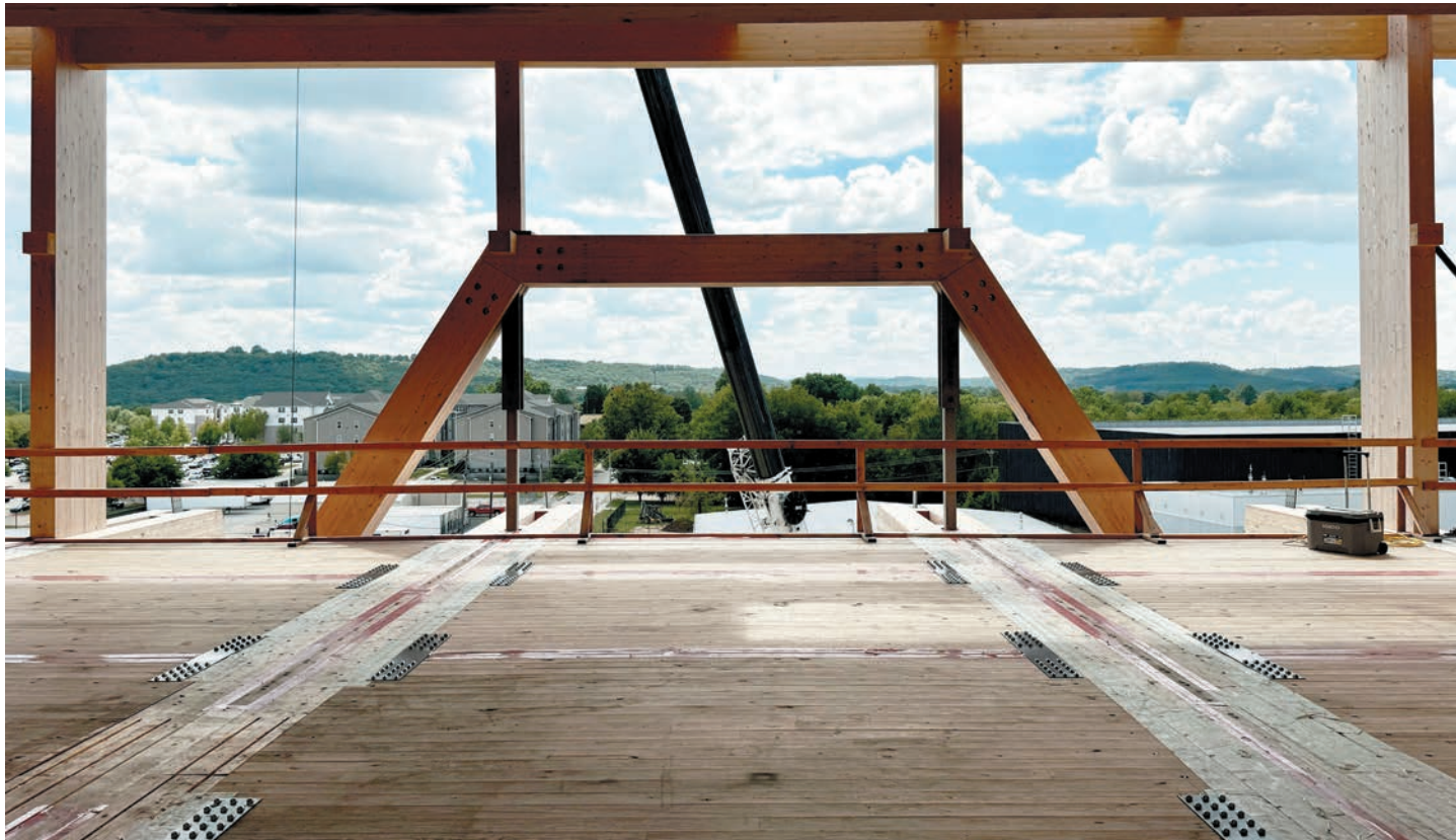
Above, a view of the top of the queen post truss, a key to the design of the Anthony Timberlands Center, during construction. Photo by Modus Studio. Below, a diagonal member of the queen post truss is visible through windows on the top level. Photo by Tim Hursley.
