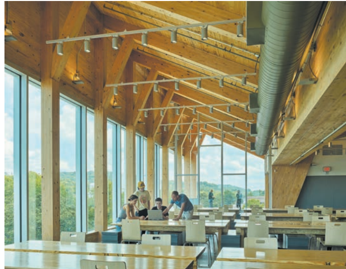
The top-level studio features an angled ceiling formed from cross-laminated timber (CLT) panels and glue-laminated beams. The studios on the top two levels are furnished with CLT desks designed by Fay Jones School students. Photo by Tim Hursley.
