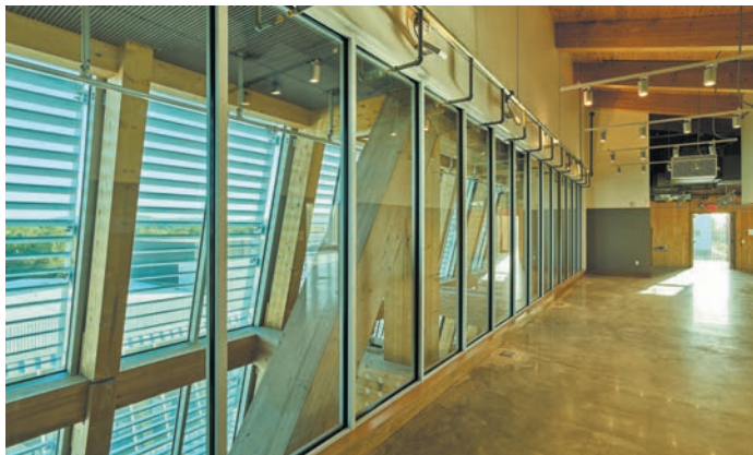
Above, a view of the top of the queen post truss, a key to the design of the Anthony Timberlands Center, during construction. Photo by Modus Studio. Below, a diagonal member of the queen post truss is visible through windows on the top level. Photo by Tim Hursley.
