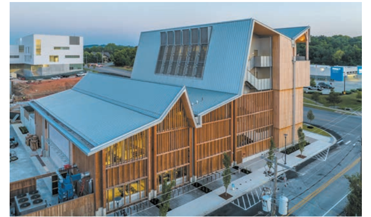
This view looking northwest shows the cascading metal-clad roof. Photo by Tim Hursley.
