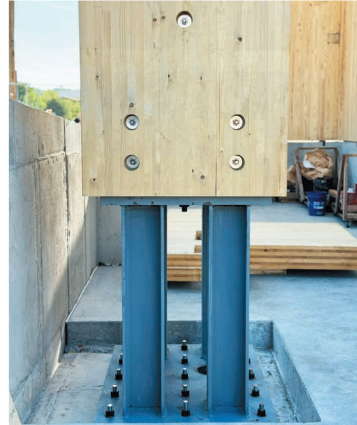
A mass timber column in the fabrication lab rests on a steel pedestal that was later enclosed in a concrete base. Photo by Modus Studio.
