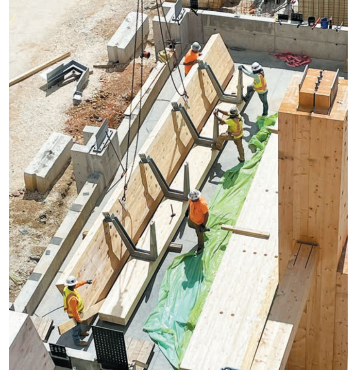
Workers form one of the two "canoe" gutters for the center. Photo by Modus Studio.
