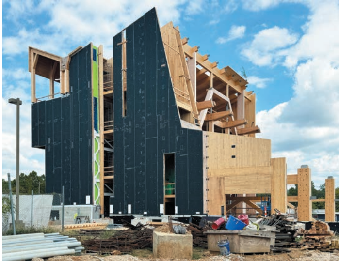
The building starts to take shape as mass timber pieces are put into place. Photo by Modus Studio.
