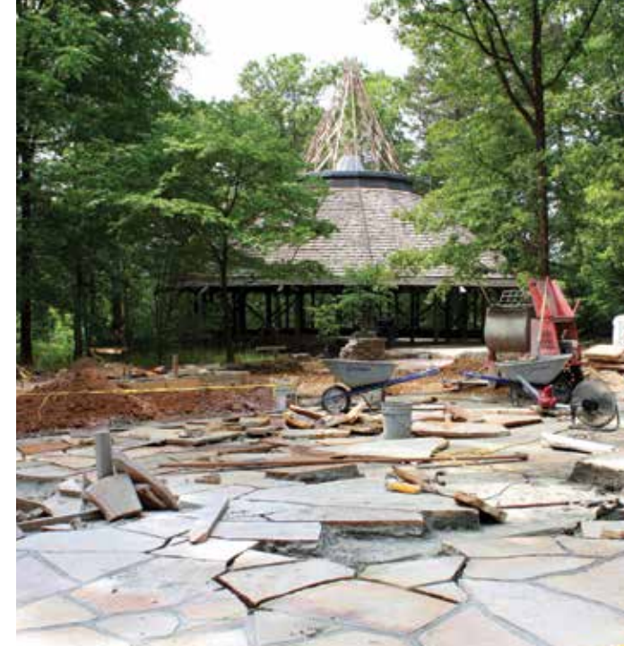
A flagstone terrace is installed in front of Garvan Pavilion.
