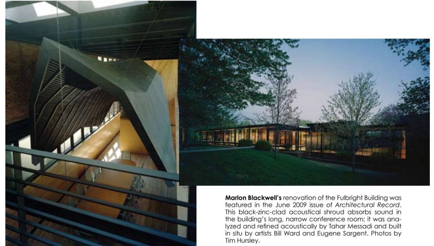
**Marlon Blackwell's** renovation of the Fulbright Building was featured in the June 2009 issue of *Architectural Record*. This black-zinc-clad acoustical shroud absorbs sound in the building's long, narrow conference room; it was analyzed and refined acoustically by Tahar Messadi and built in situ by artists Bill Ward and Eugene Sargent. Photos by Tim Hursley.
