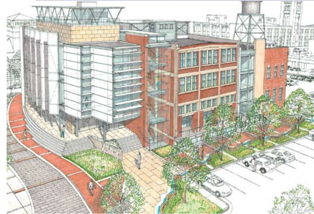
A landscaped plaza links the Arkansas Studies Institute with the existing library building.
